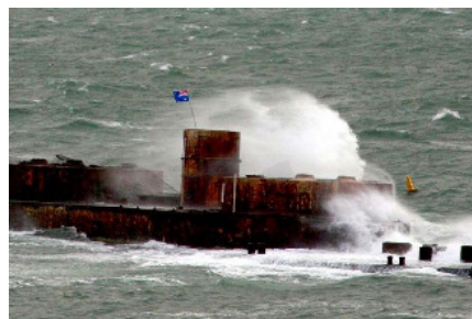
Federal 'protection' fails to stop the HMVS Cerberus from rusting away
