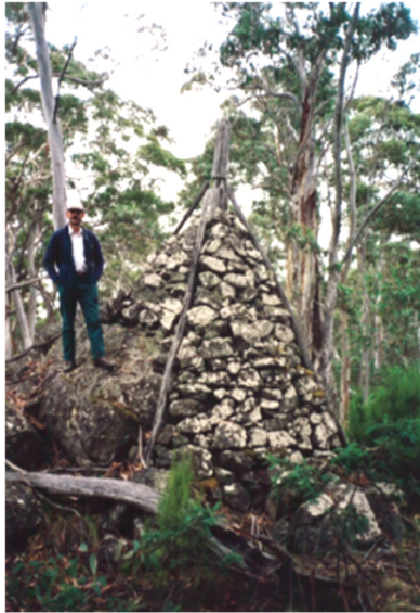
In 2004 a survey group from RMIT followed in the footsteps of Black and Allan, and repaired many of their original stone cairns ( click here )
